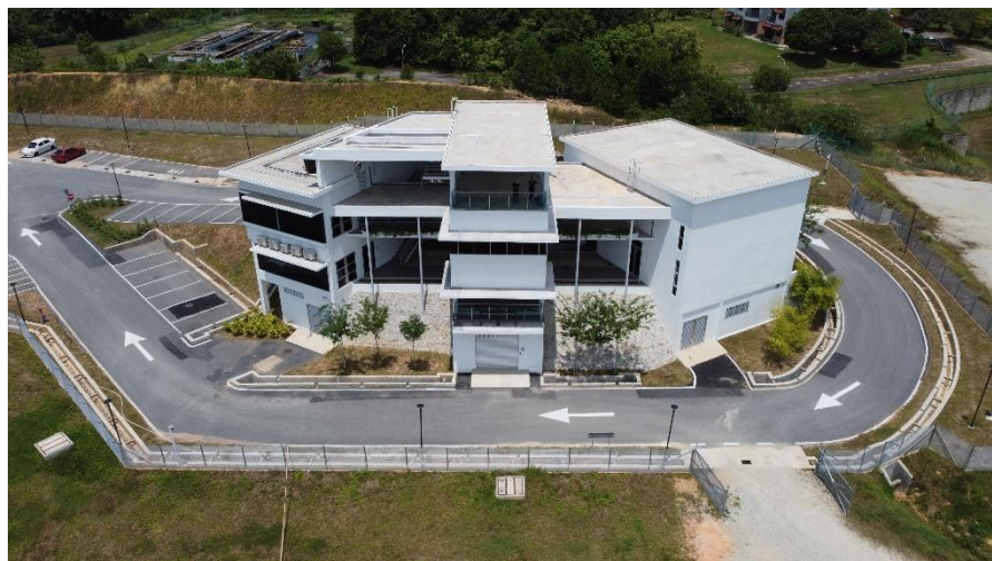
Sumber: : UiTM Energy & Facilities Sdn. Bhd. (2022); LSSPV Gambang, Pahang
