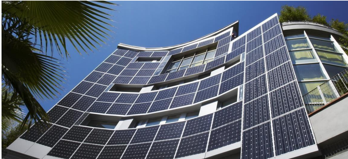
Sumber: Mapsolar Group (2020); Rainscreen Cladding - Solar PV facade - 25kW photovoltaic panelsystem, F.LLi Cava Building, Italy
