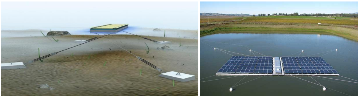
Sumber: SPG Solar Inc. (2010); Anchoring and mooring system, Far Niente Winery, Oakville, California
